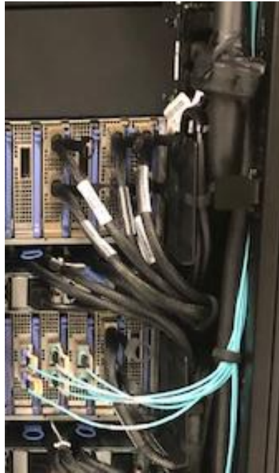
Figure 29: Coupling Cabling with Hook-and-Loop Fasteners
