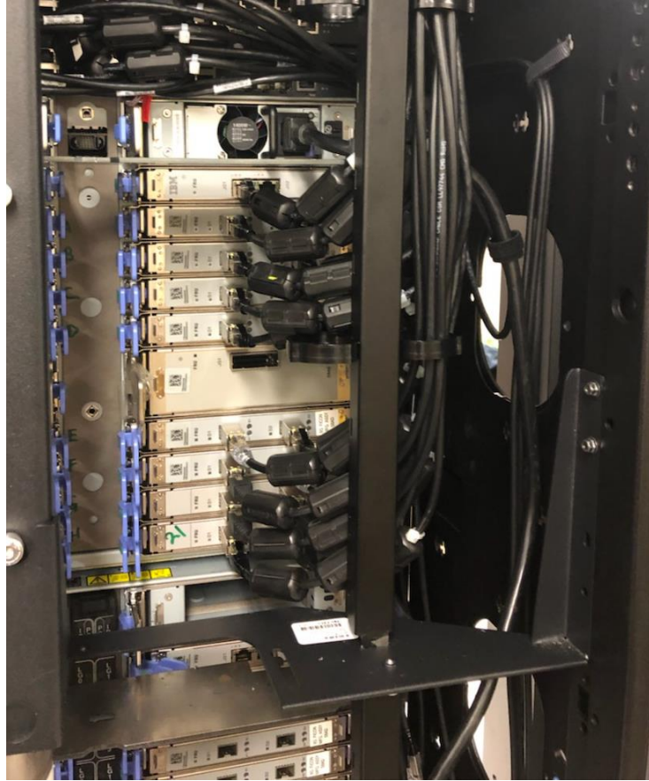
Figure 30: OSA Cables in Mini-Spine
