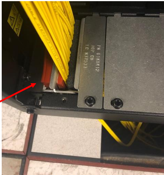
Figure 17: Fiber Optic Cables in Strain Relief Clamp for Bottom Exiting System
