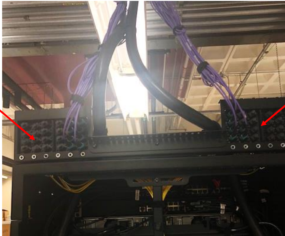
Figure 27: Fiber Quick Connect in Top Exit Cabling Enclosure (FC 7898)
