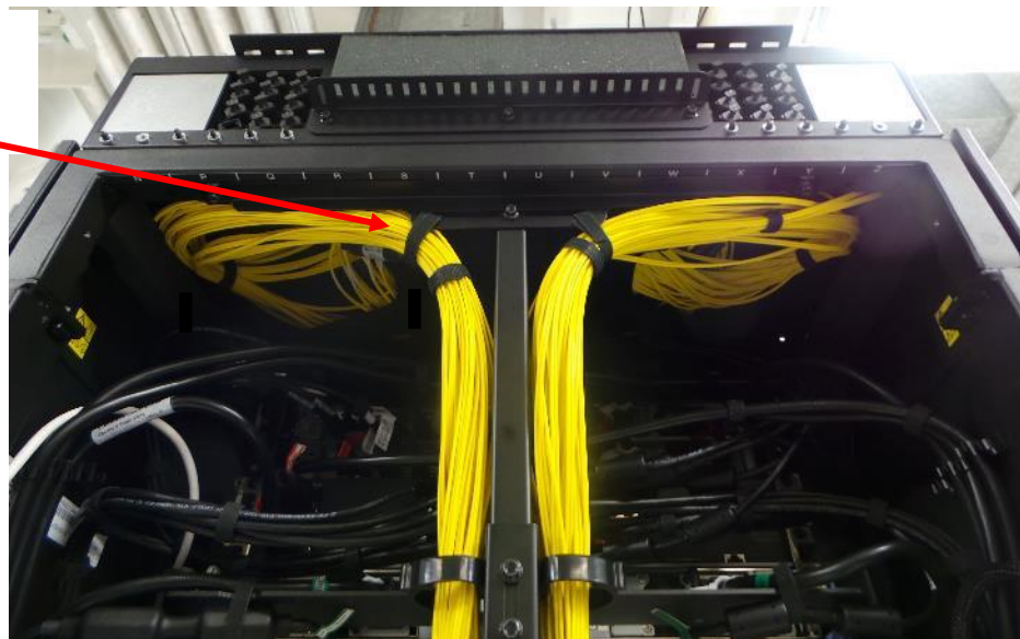
Figure 15: Horizontal Cable Support
