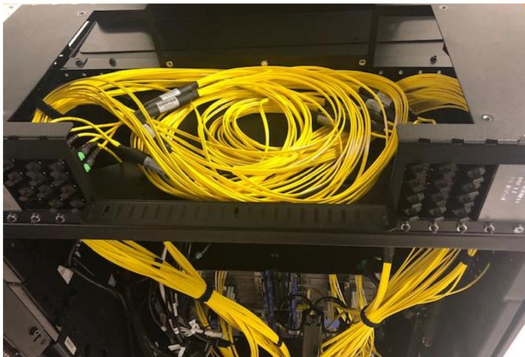
Figure 28: Fiber Cables in Top Exit Cabling Enclosure
